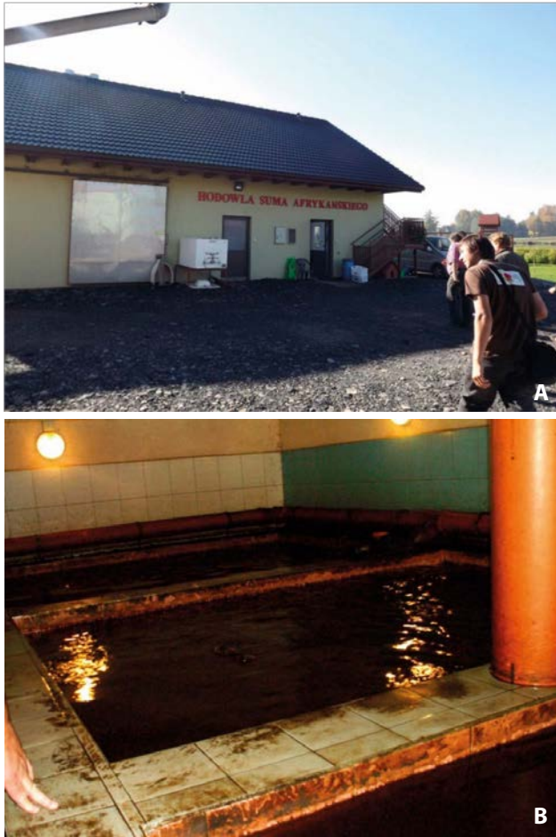
Fig. 5. Exterior (A) and interior (B) of originally agricultural building which was adapted and rebuilt a farm with intensive rearing of African sharptooth catfish (firm „Krolestwo ryb”) in Pielgrzymowice in Poland. Photo by J. Kouřil
